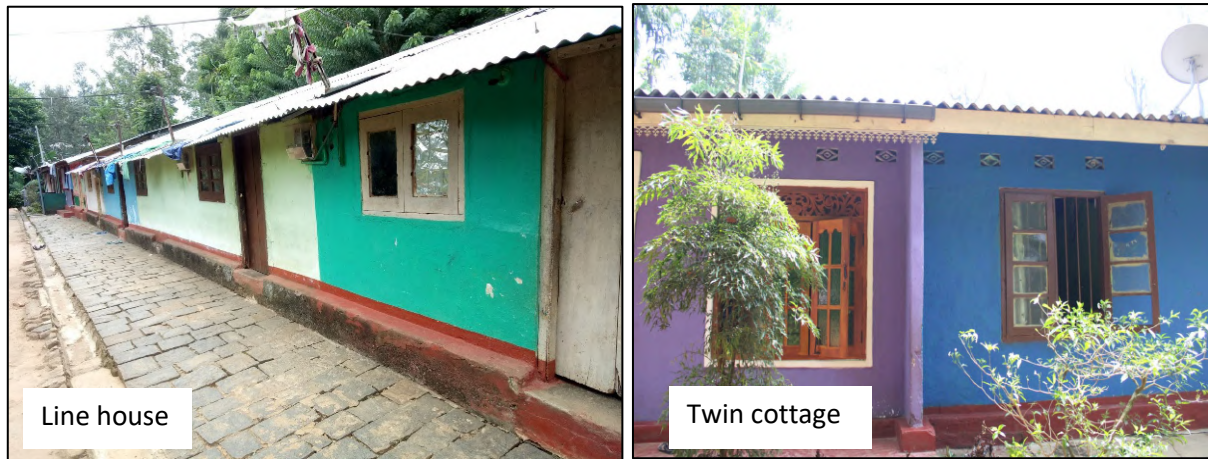
Figure 3 The housing structures in the Sarnia community
